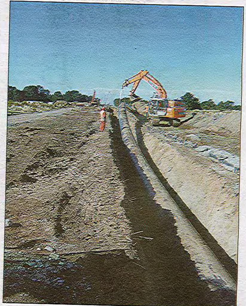
Dormer Construction using its diggers to lay pipes for the Waimakariri District Wastewater Outfall Connecting Pipeline.
